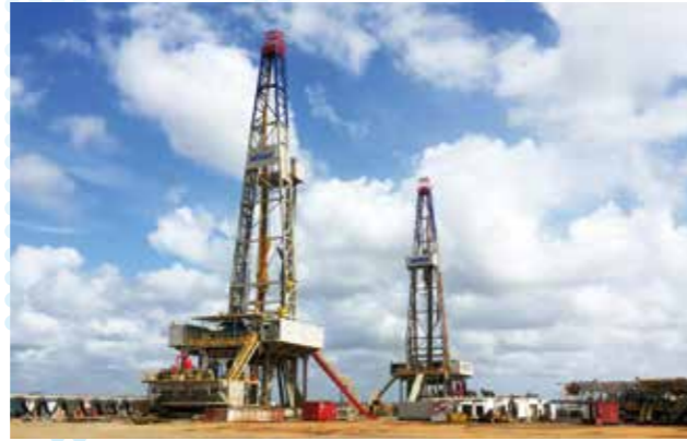
Drilling and Workover Engineering Technology Services
