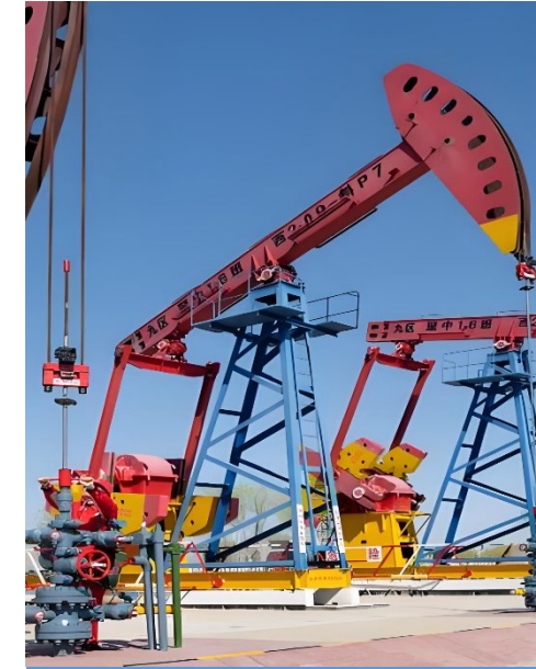
Construction of Oil Production System
