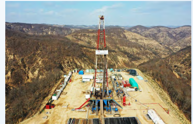
Northern Shaanxi Tight Oil Drilling Platform
