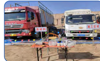
Oilfield Wastewater Reuse
