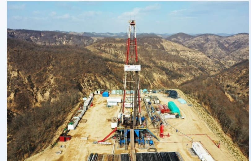
Northern Shaanxi Tight Oil Drilling Platform
