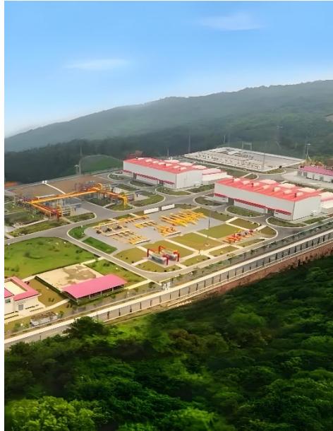
Surface Facility Support Systems
