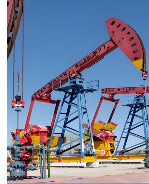
Construction of Oil Production System
